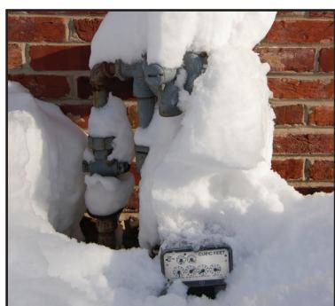
The major snowstorm that affected the area in late January caused snow drifts while snow removal operations created snow mounds around homes and businesses. The WMGLD reminds customers that heavy snow placed against the building's natural gas meter can cause damage to the gas regulator and overflow valve, causing it to
