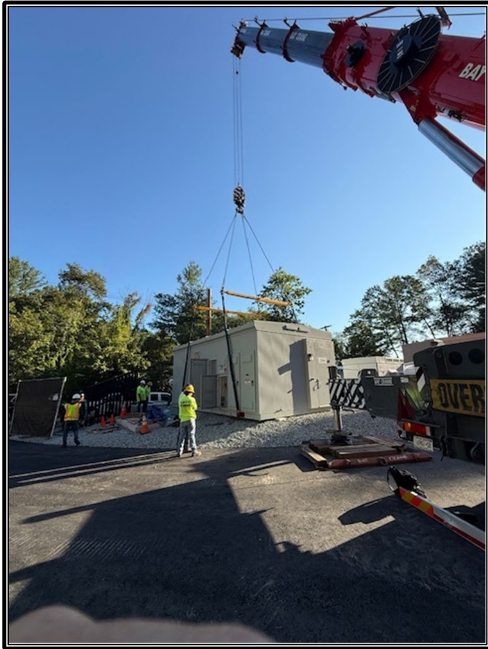
Switchgear Installation Picture 2
