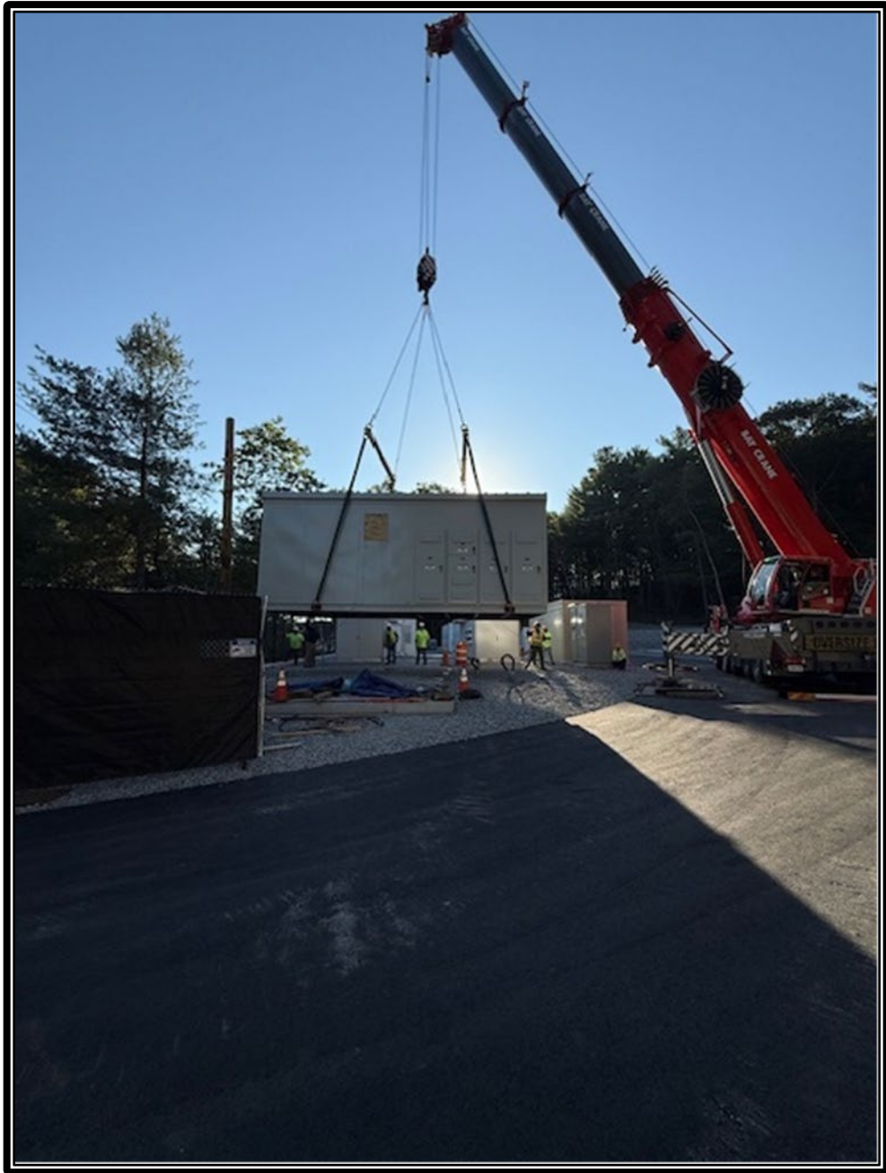
Switchgear Installation Picture 1
